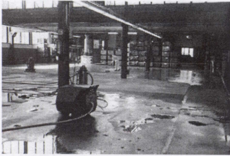
Final Cleaning plus coating.
